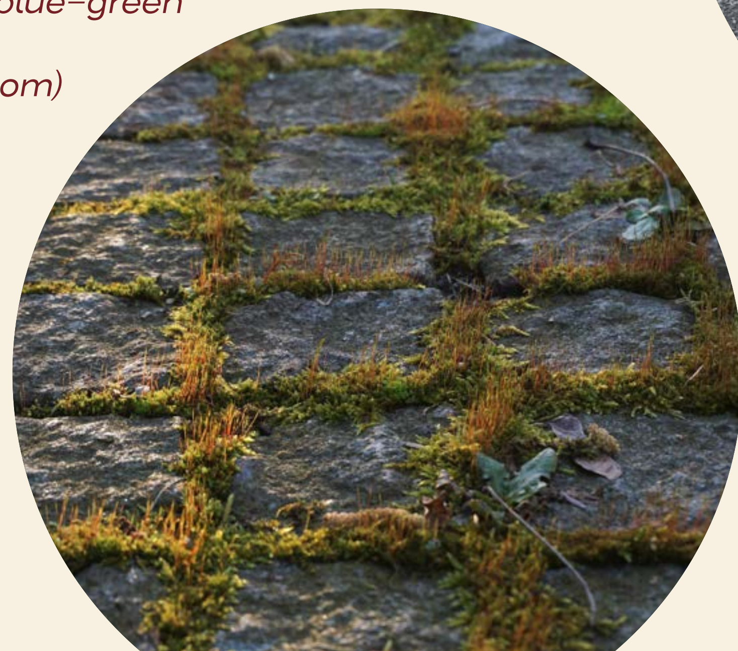
Permeable gravel surfaces (photo: Alabama Extension, openverse.org, licence CCO 1. 0.)
